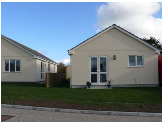
St Minver CLT Self-Build Development, 2008.
